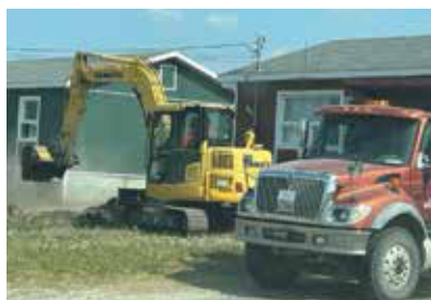
Road and Walkways Operators assisting Water Department
